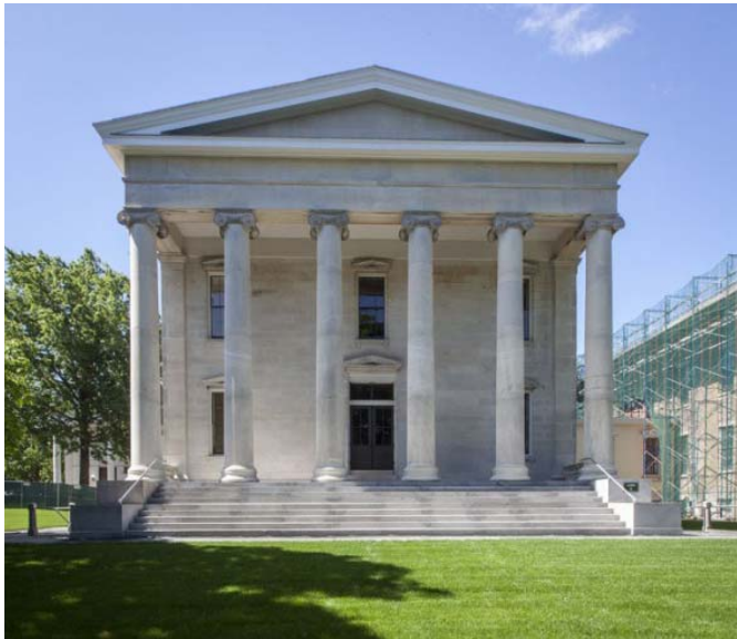
Snug Harbor Building E's exterior restoration
